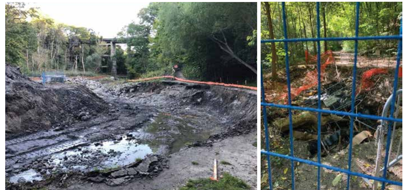
Work Underway on Yellow Creek (Oct. 2024)
